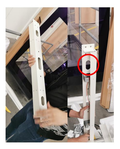
Remove the covers of the mounting arms and feed the USB extension cables through to the end and fix in place with the screws provided.
